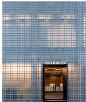
Glasbrick facade | Renzo Piano Architects, Flag ship store Hermès Tokyo
