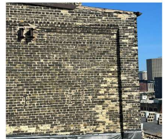
Brick condition on the rooftop
