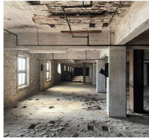
Reinforced concrete supporting structure
