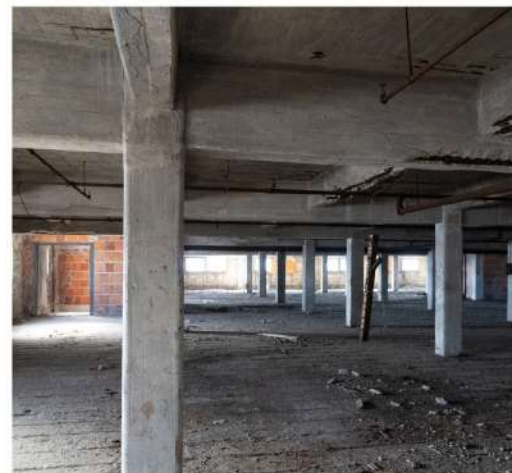
Reinforced concrete supporting structure
