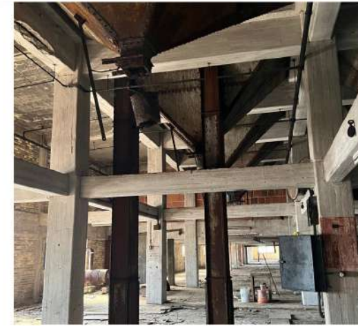
Silo elements towards supporting structure
