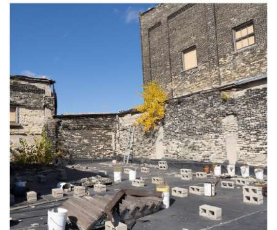
Brick condition on the rooftop
