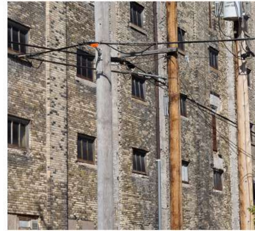
Brick cladding on the east facade
