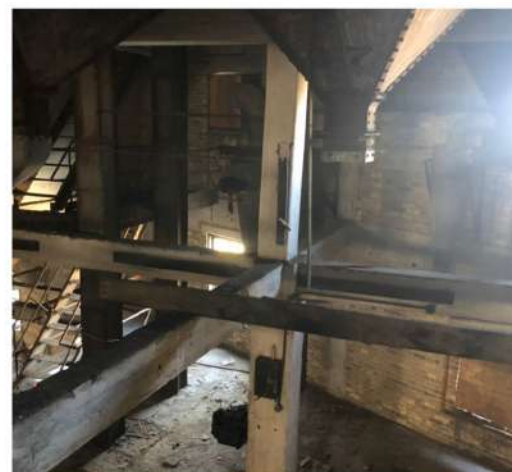
Bottom part of the silo construction
