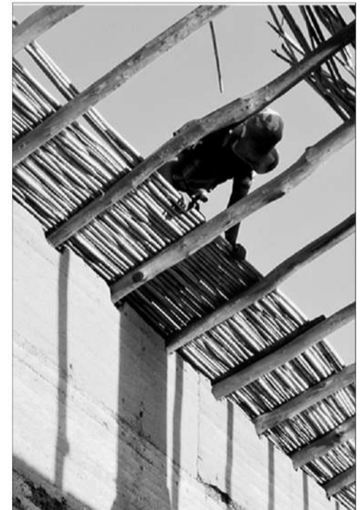
Wooden structure roof
