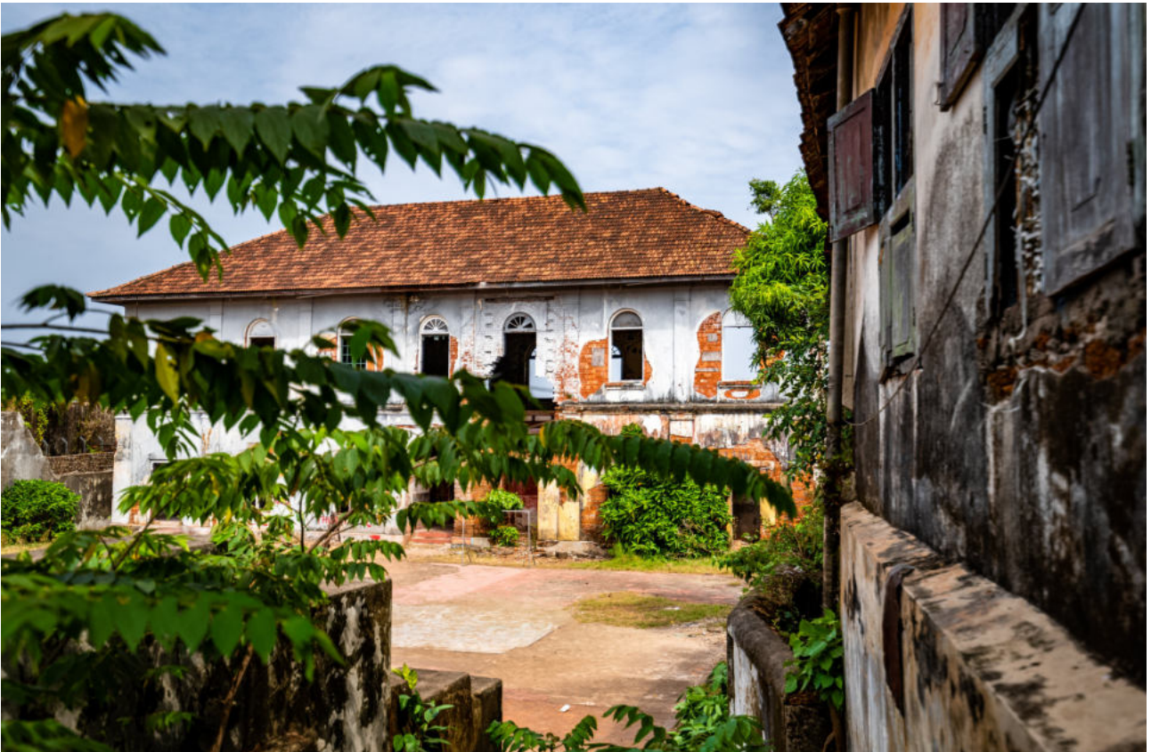
Figure 5-5: Abandoned colonial era structure. Source: author.
